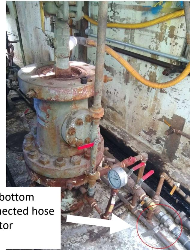
Note: Red circle at bottom right indicates connected hose for corrosion inhibitor treatment
