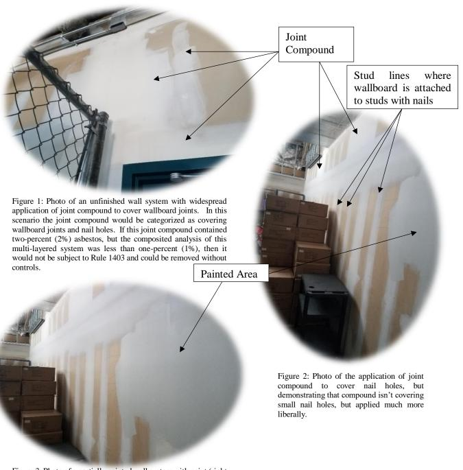
Figure 3: Photo of a partially painted wall system with paint (right side) covering joint compound and concealing where it was applied to the wall system
