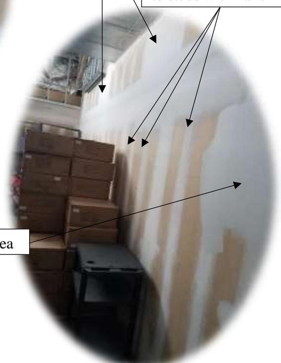
Figure 2: Photo of the application of joint compound to cover nail holes, but demonstrating that compound isn't covering small nail holes, but applied much more liberally.
