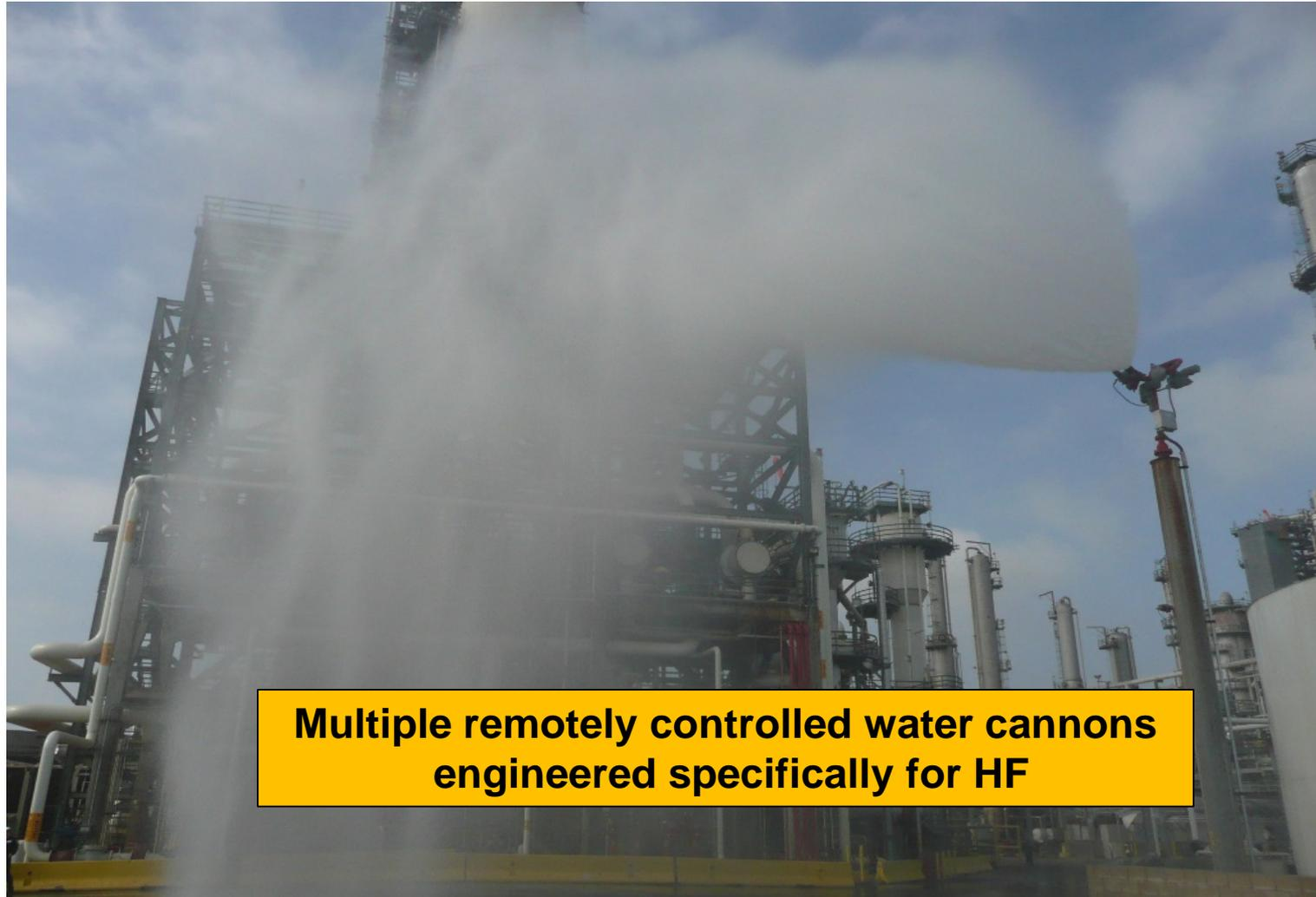
**Multiple remotely controlled water cannons
