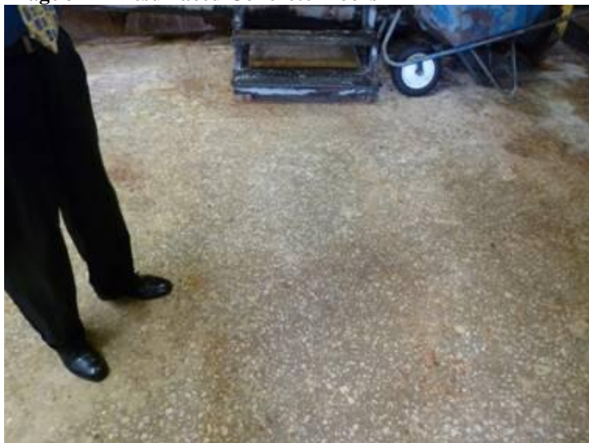
Image 3-1 – Resurfaced Concrete Floors
