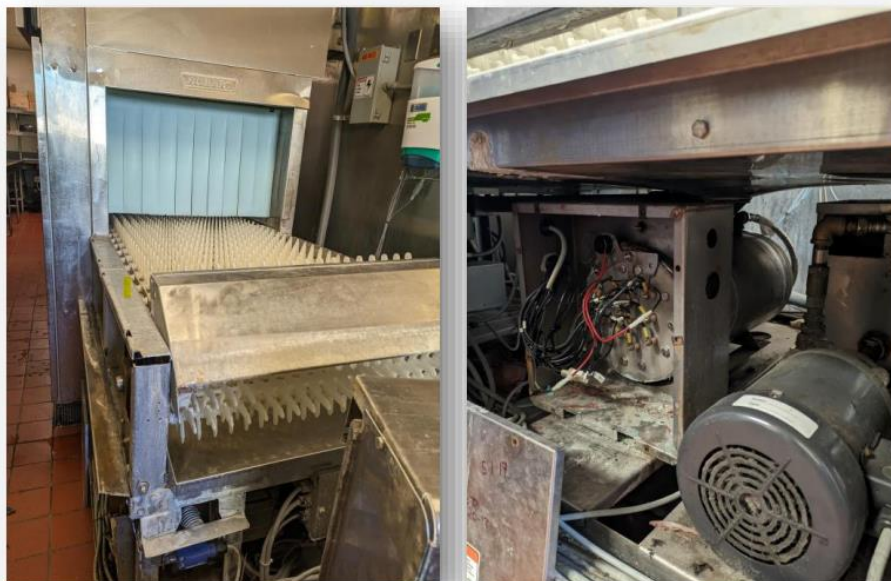
Figure 2-4. Examples of Dishwashing Unit (Left) and Electric Booster Heater (Right) Zero-Emission Co-Benefits
