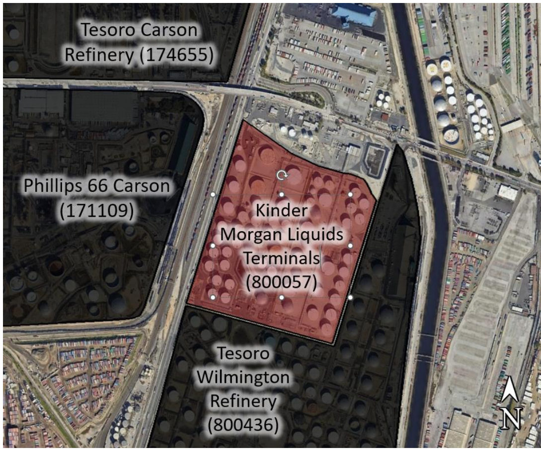
Figure 2-17: Kinder Morgan Liquids Terminals Facility
