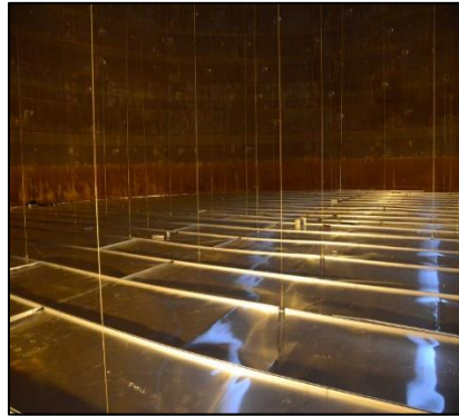
Figure 2-4: Cable Suspended Roof
