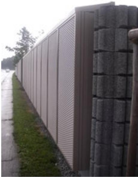
**Figure 2: Filter panel installed on a noise barrier for the SPAS study. (Magistrat Klagenfurt 2011)**
