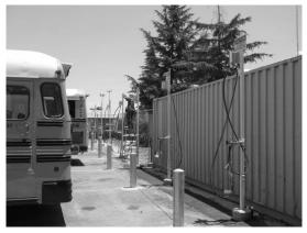
Figure 1: Time-Fill Posts Allows Beaumont USD to Fill 8 Buses Overnight
