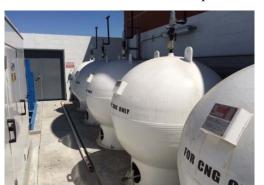
Figure 21: CNG Storage Spheres
