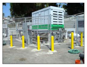
Figure 1: Compressor with Catwalk
