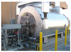
Figure 1: TVRWRF Noxtech® Reactor
