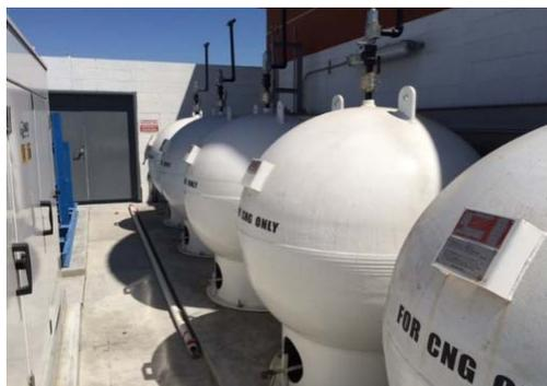
**Figure 21: CNG Storage Spheres**
