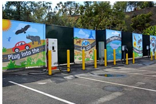
**Figure 1: Los Angeles Zoo, DC Fast Charger and Level 2 EVSE (electric vehicle supply equipment)**
