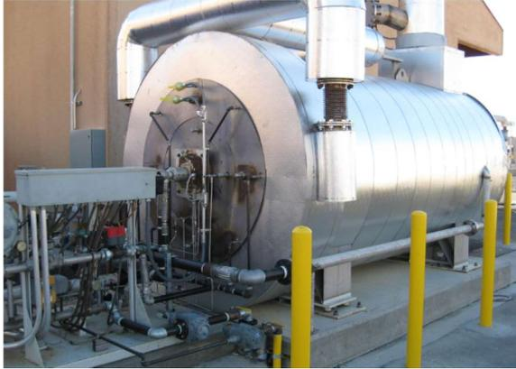
Figure 1: TVRWRF Noxtech® Reactor
