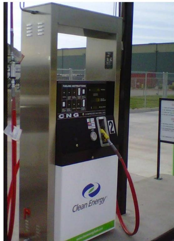
**Figure 2: CNG Dispenser installed at Agua Mansa LNG Station**
