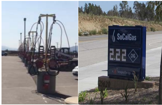
Figure 2: Time-fill Posts Figure 3: Public Signage
