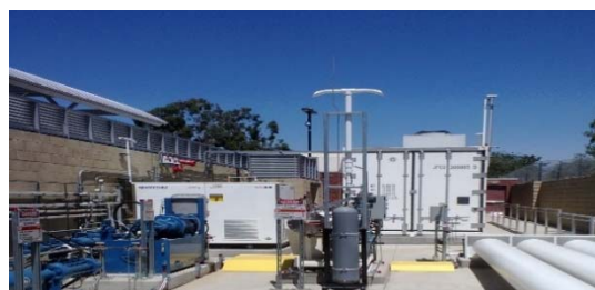
Figure 1: CSULA's H 2 Station interior (from left to right): high pressure compressors, H 2 chiller, 350 bar compressor, electrolyzer, 350 bar storage banks, visitor gallery
