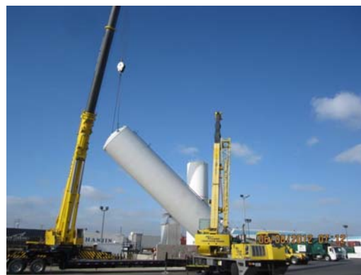
Figure 1: LNG Tank Installation
