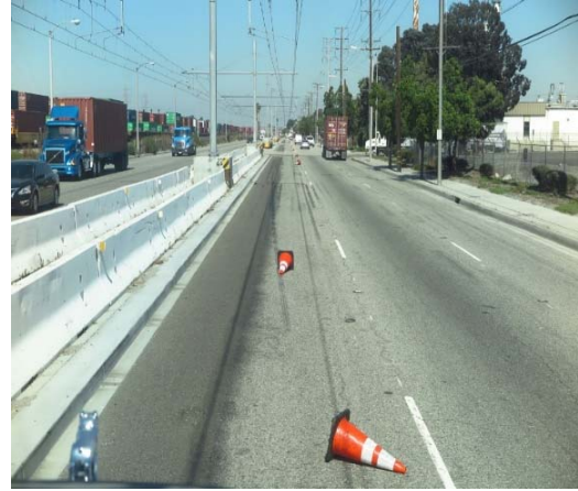
Figure 17: eHighway Infrastructure on Alameda Street
