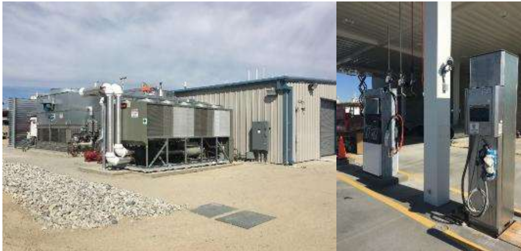
Figure 7: SunLine Transit Agency Onsite Hydrogen Fueling Infrastructure
