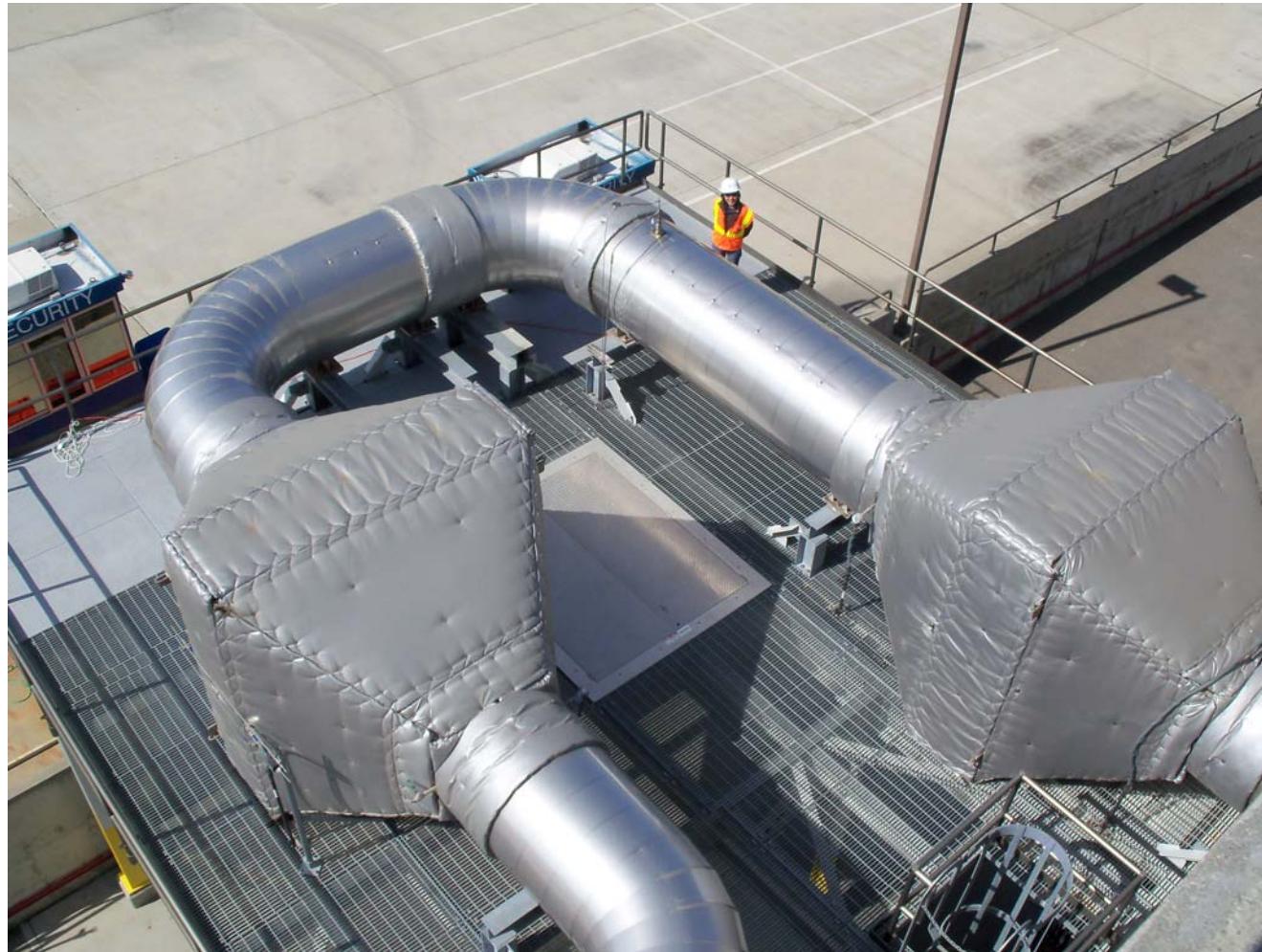
Figure 2-4: Cat Ox/SCR Platform Installation
