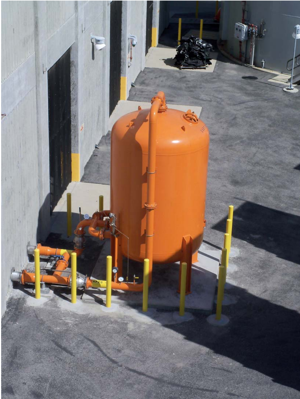
Figure 2-3: Digester Gas Cleaning System
