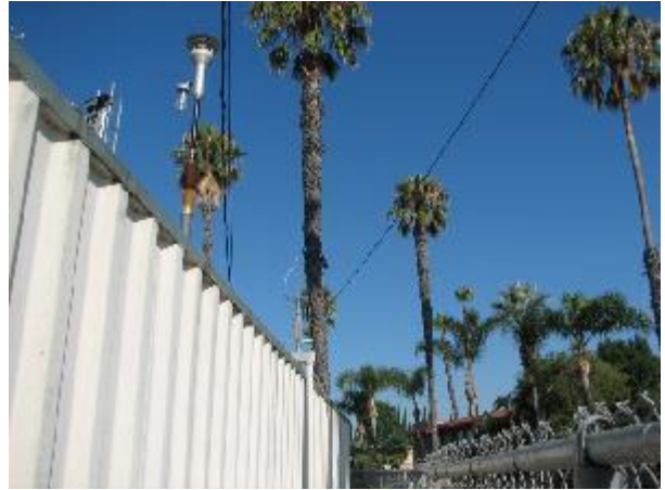
Looking at the probe from the East.
