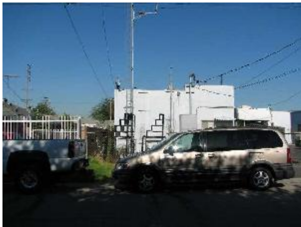
Looking at the probe from the South.
