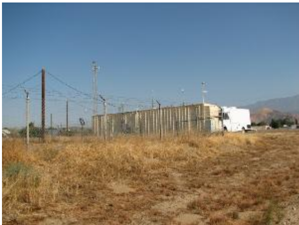
Looking at the probe from the South.
