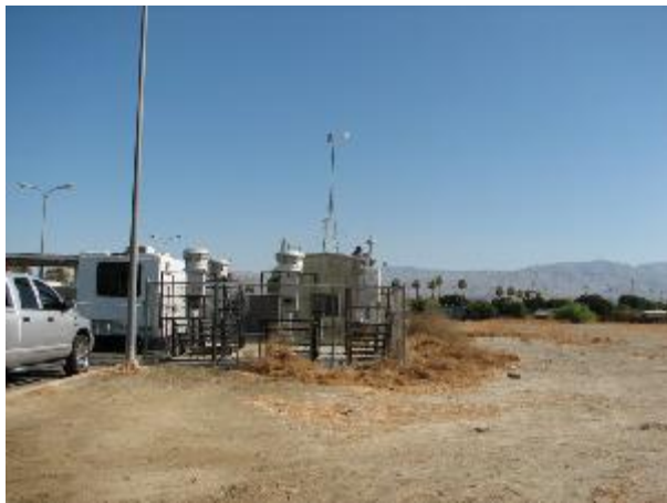
Looking at the probe from the South.
