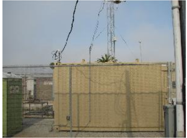
Looking at the probe from the East.
