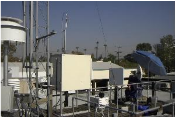
Looking at the probe from the South.
