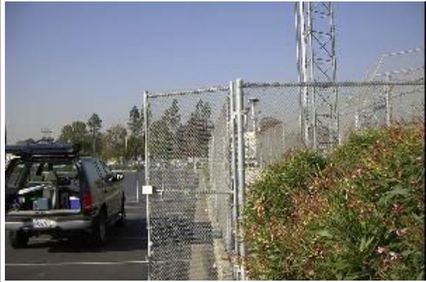
Looking at the probe from the East.
