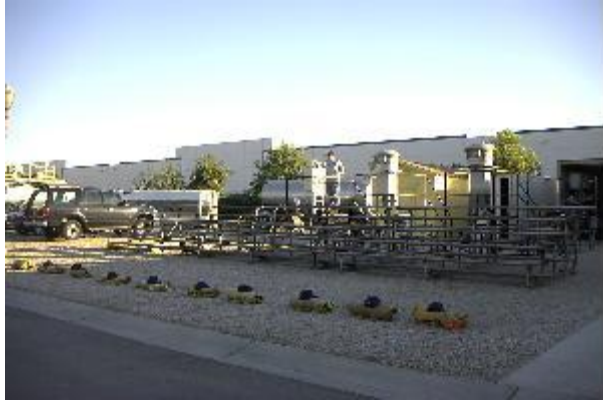
Looking at the probe from the North.
