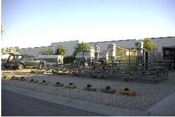
Looking at the probe from the North.
