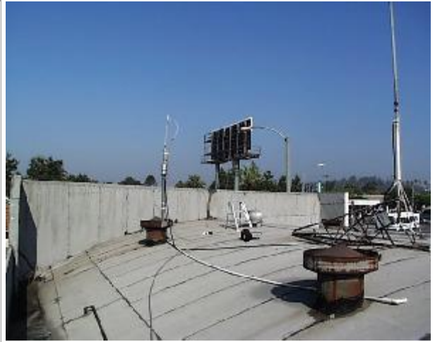
Looking at the probe from the East.
