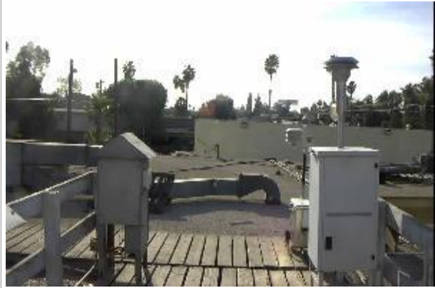
Looking at the probe from the East.
