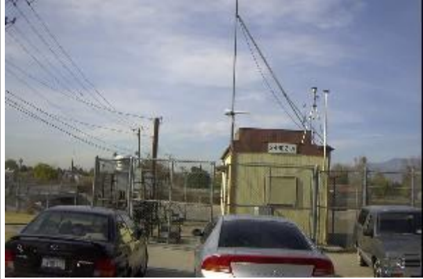
Looking at the probe from the East.
