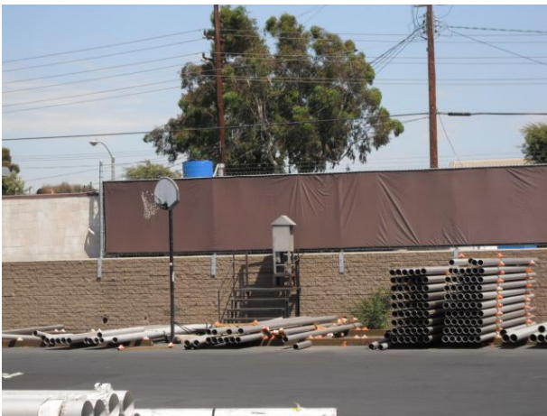
Looking South toward the probe.
