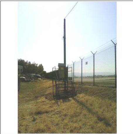
Looking South toward the probe.
