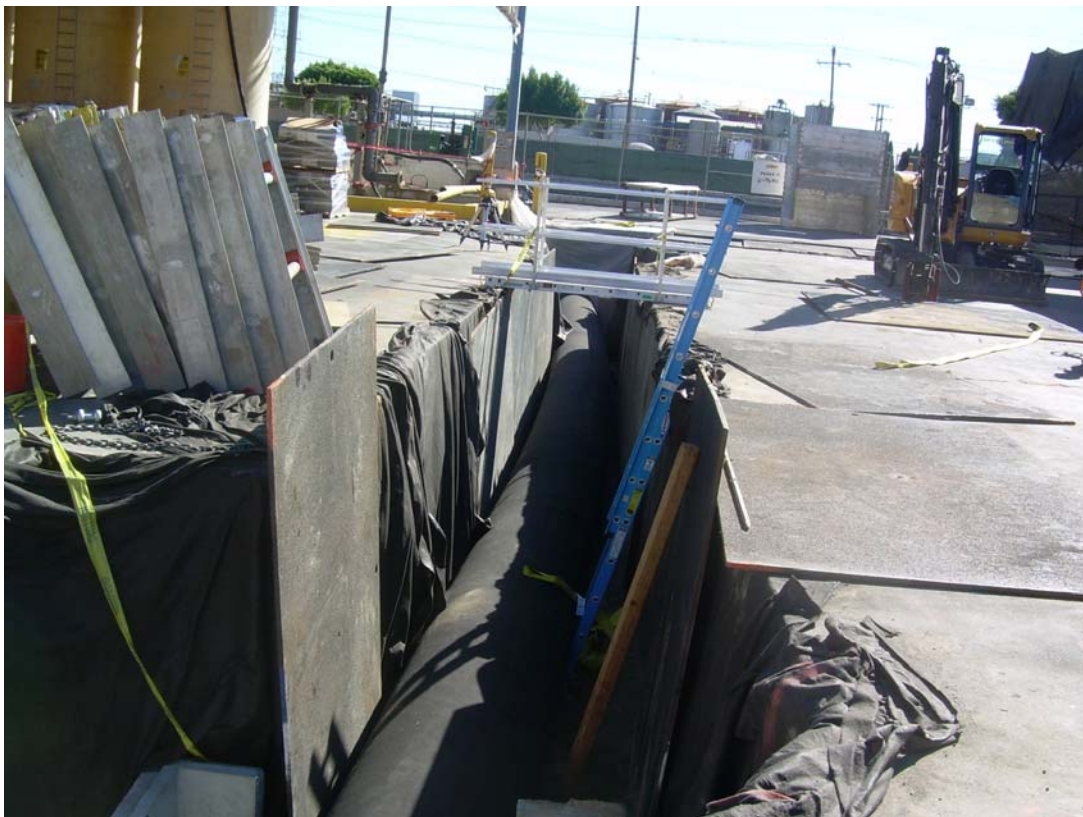
Figure 3-2 Current Replacement of Storm Water Piping
