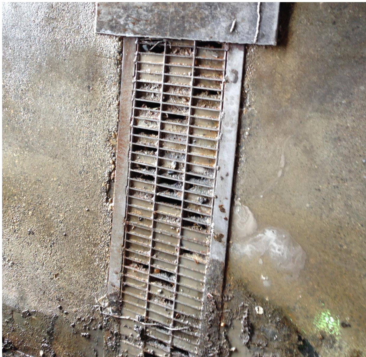
Image 3-2 Clogged Wastewater Channel
