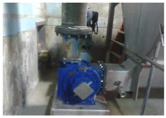
Typical grinding equipment observed at a local rendering facility.
