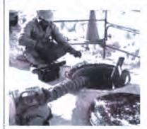
Continuous ventilation and leading are critical in any confined space with a harmful atmosphere.
