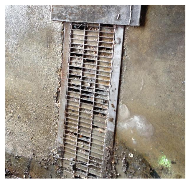
Image 3-2 Clogged Wastewater Channel
