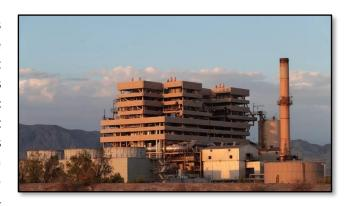
electric power plant<sup>1</sup>. Typically, these power plants operate by burning fuel in a furnace to generate heat that is used in a boiler to produce steam. The steam flows into the turbine and spins the blades inside a turbine, which is connected to a generator to create electricity.
