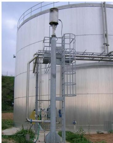
**Figure 3-1. Non-Hydrogen Clean Service Flare (LPG Flare)**
