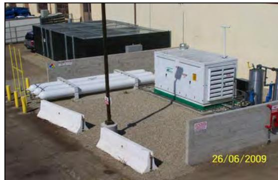
Figure 1: CNG Station Filter Dryer & Compressor at City Yard
