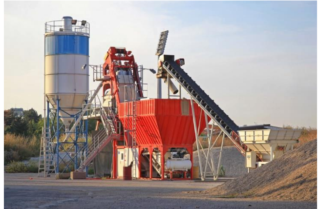
Figure 5f-1: Concrete batch plant
