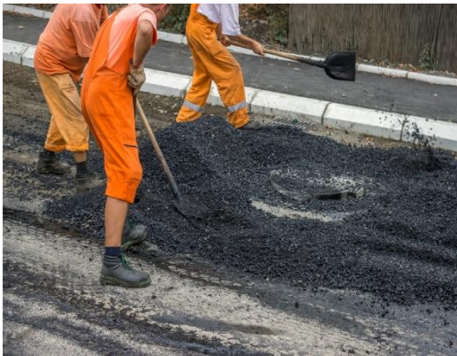
Figure 5f-2: Asphalt being used for paving
