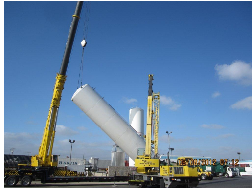
Figure 1: LNG Tank Installation
