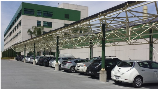
Figure 2: SCAQMD solar carport featuring upgraded EVSE
