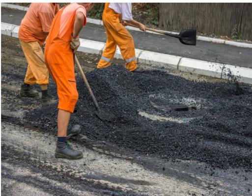
hot mix asphalt. Smoke is released from the hot oil and the hot mix asphalt and can cause odor nuisances.
