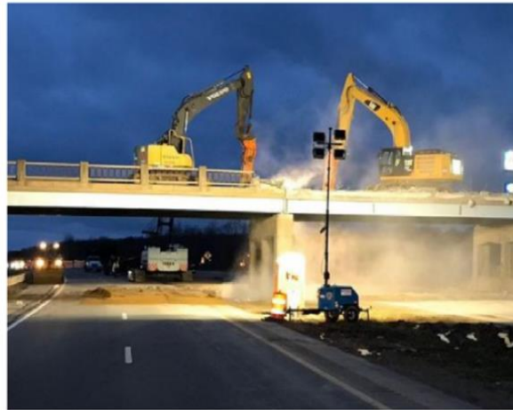
Figure 1-4 Bridge Demolition Activity Over a Large Roadway
