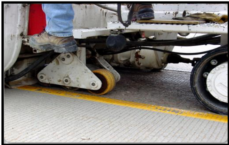
Figure 2-6: Slurry Recovery Vacuum on Texture Planer
