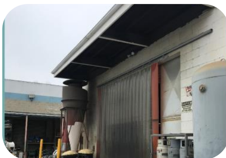
Cross-Draft Minimization Using Overlapping Strip Curtains
