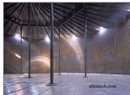
Initially, cable suspended floating roofs were estimated to decrease standing losses by 35%<sup>2</sup>, as based on results from TankESP PRO software. Emissions
