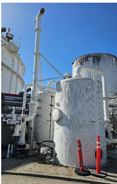
Figure 2.8 - Example of a Vapor Recovery System
