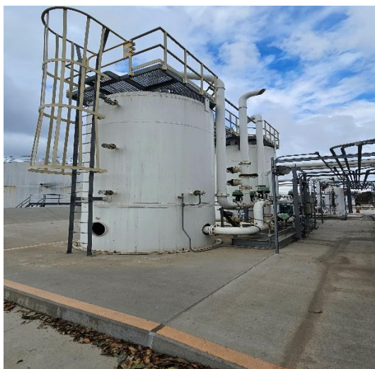
Figure 1.2 – Example of a Vapor Recovery System
