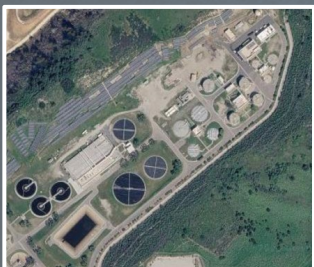
Water treatment facilities
