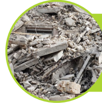
Construction and Demolition Debris Transfer Station
