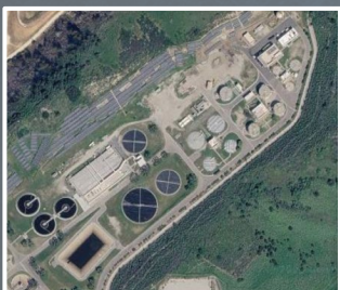
Water treatment facilities
