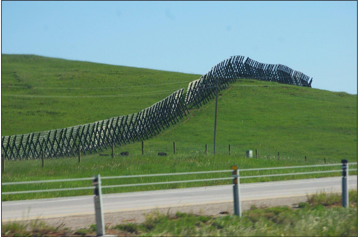
Figure 13 - Drift fence with 50% porosity
