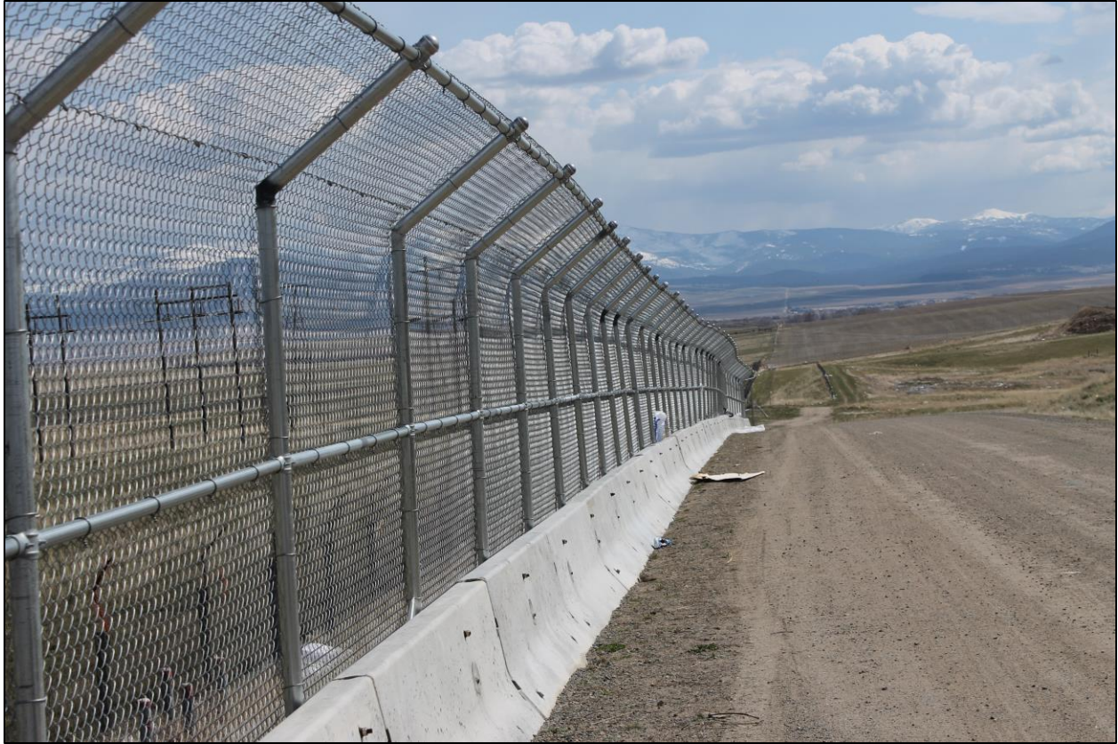
Figure 16 - Fence with 80% porosity
