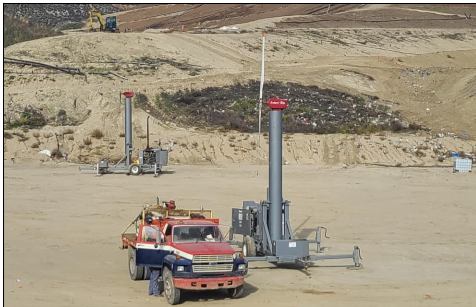
Figure 18 - Diesel-powered Orchard fans
