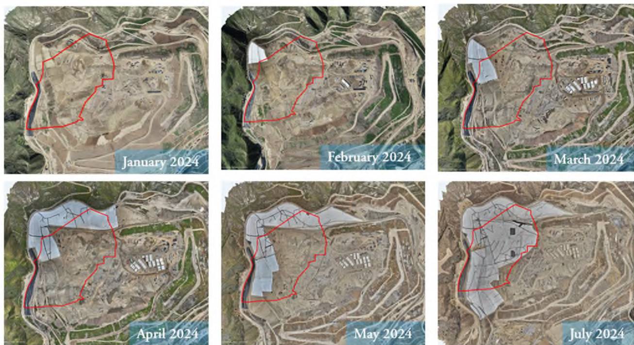
Figure 20. Aerial images of the progression of Chiquita's installation of the geosynthetic cover from January to July 2024. The red line illustrates the approximate boundaries of the data-driven reaction area.
