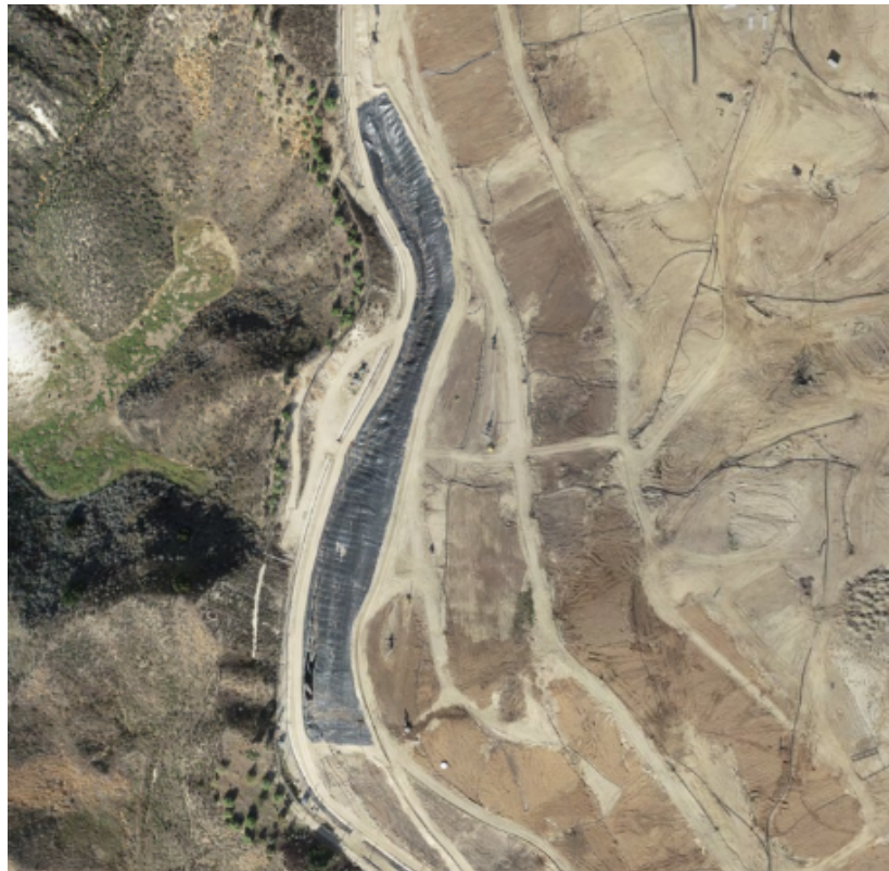
Figure 22. Aerial image of the temporary plastic cover (scrim) on the west slope of the Landfill (December 2023).
