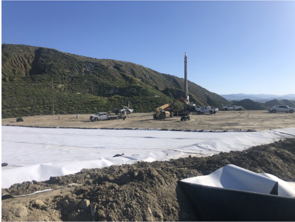
Figure 6. Picture of the installation of the geosynthetic cover at the Landfill.
