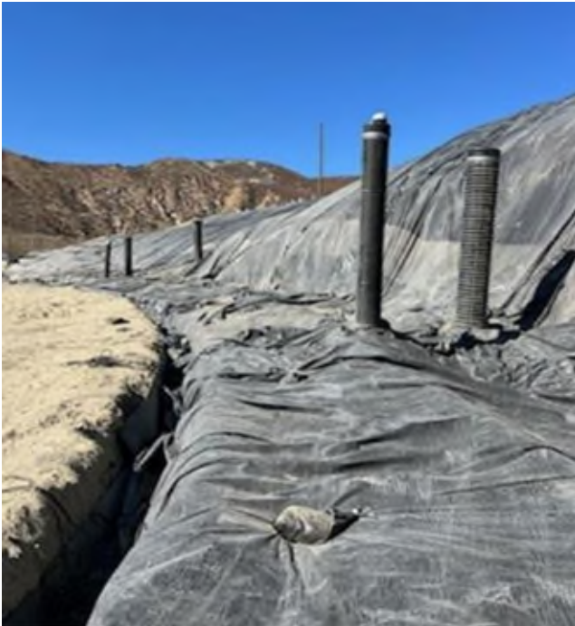
Figure 24. Images of the west slope post-excavation and installation of the new toe drain.
