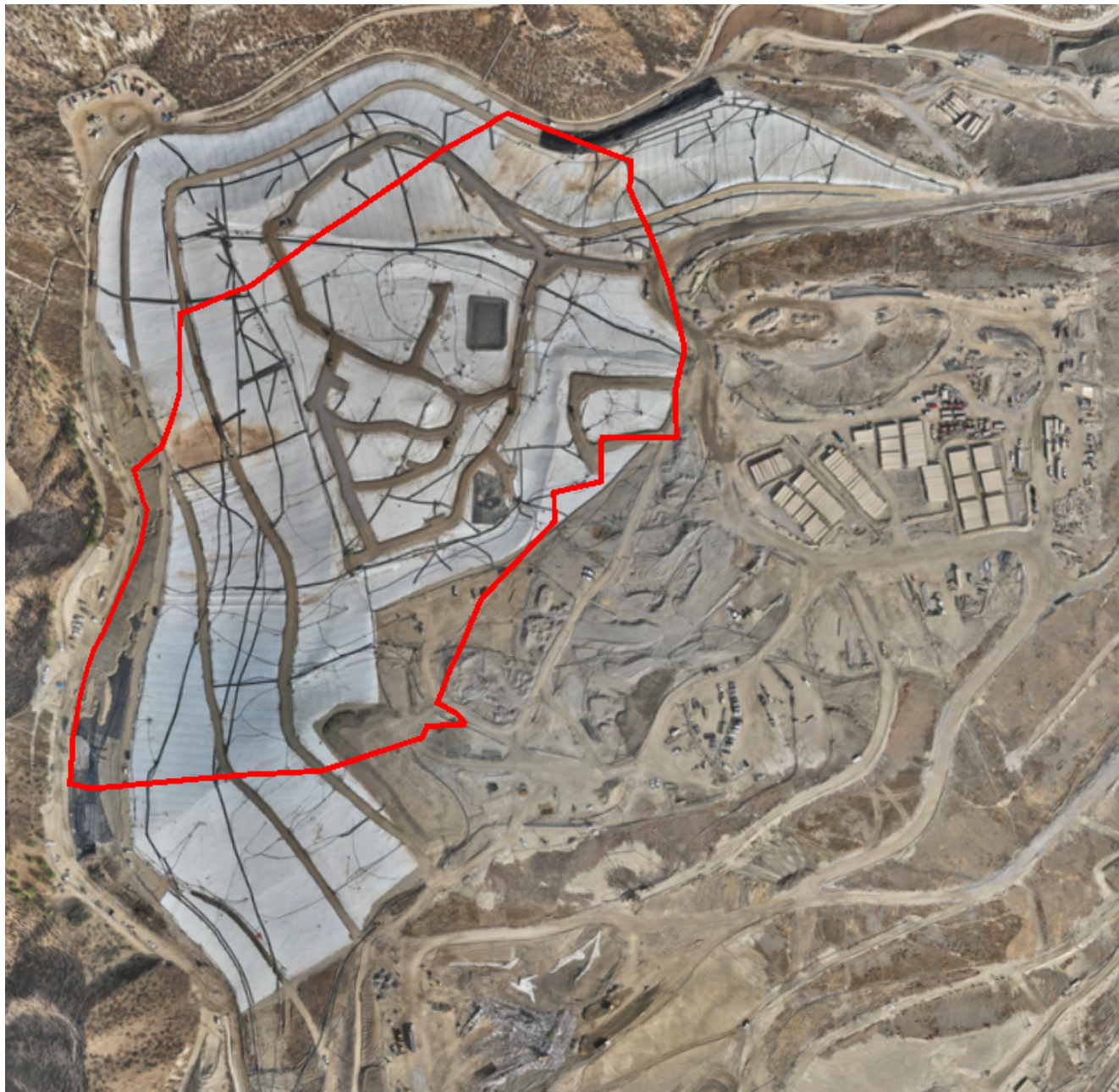
Figure 4. Aerial image of the geosynthetic cover over portions of the reaction area (approximated by the red line). Chiquita had installed approximately 41 acres of cover as of October 31, 2024.
