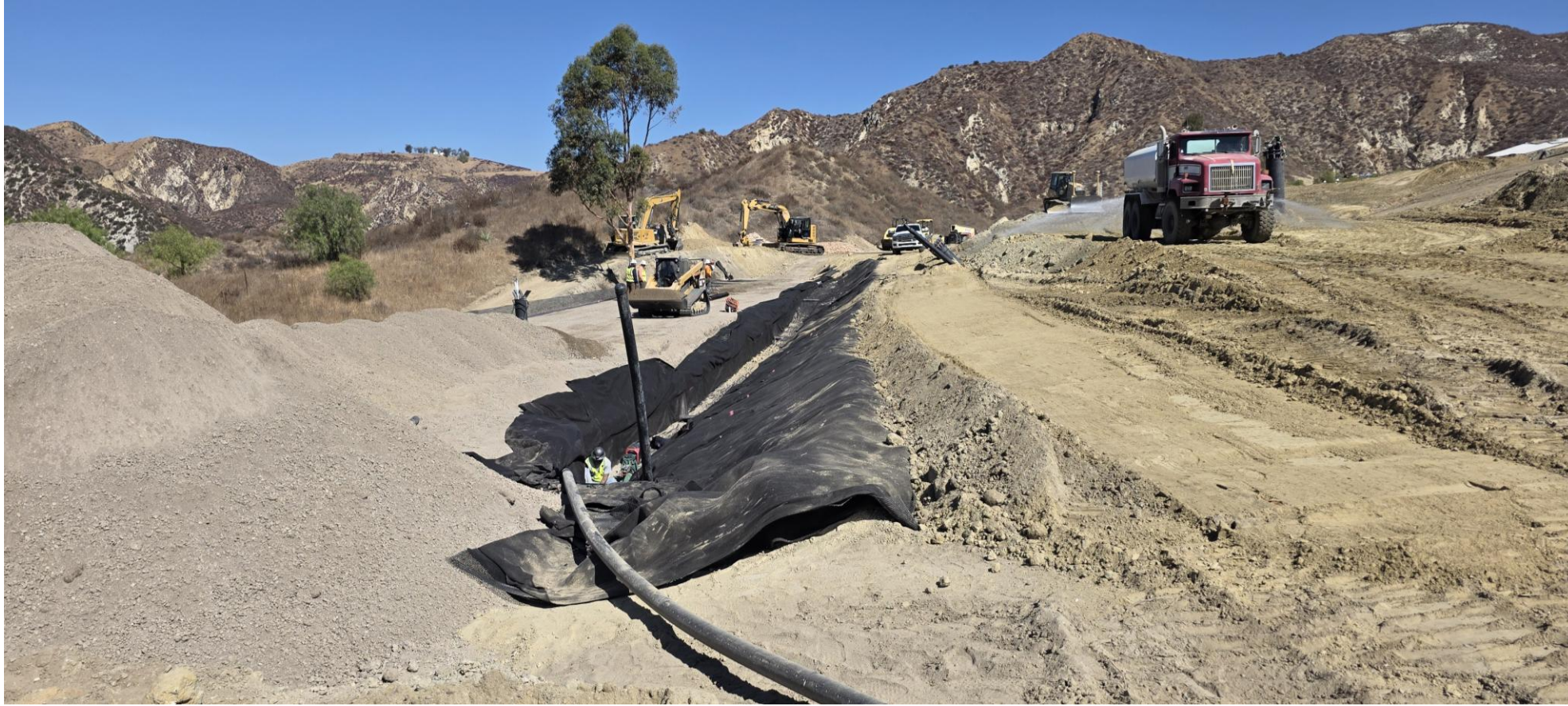
West Slope Buttress Project - Construction
