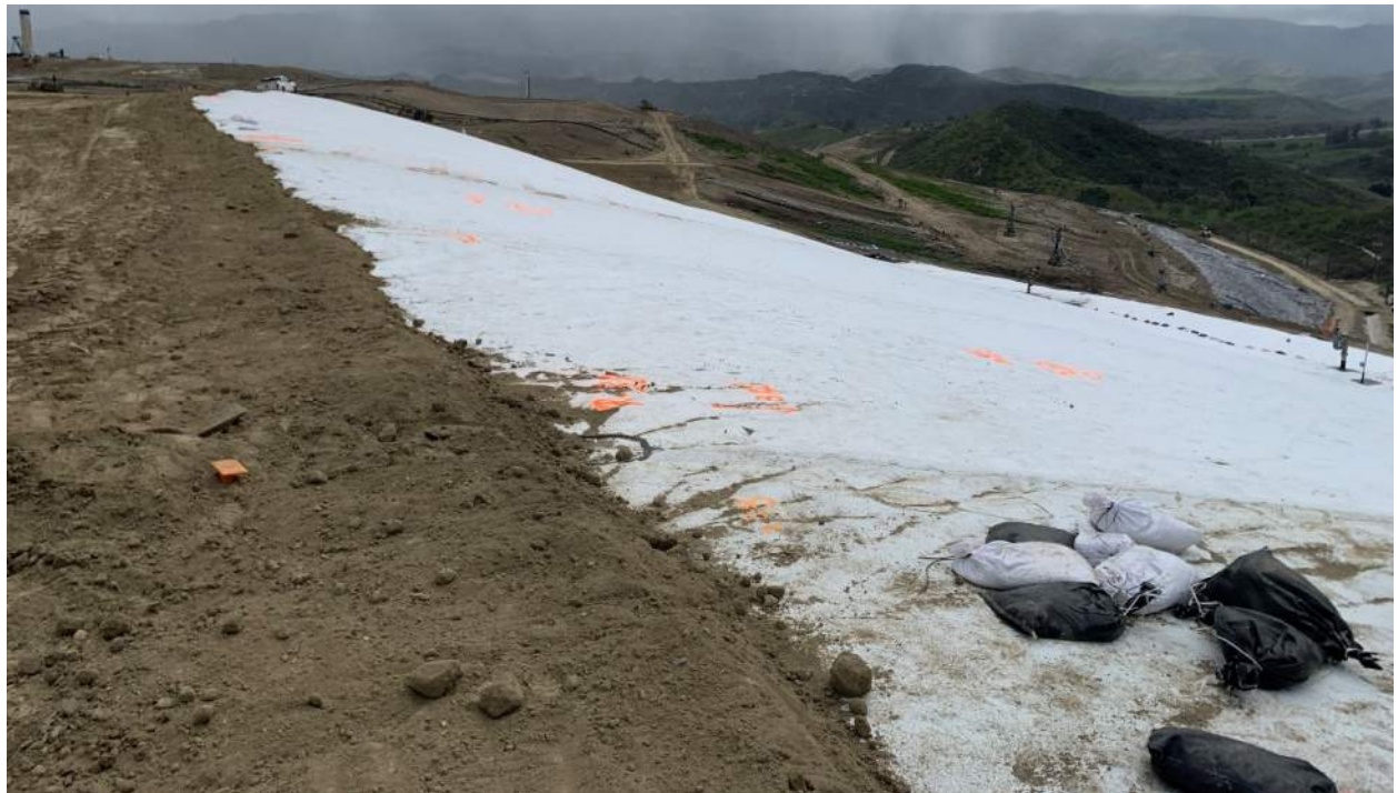
Photo #4 March 1, 2024 Top Deck Anchor Trench with Geosynthetic Cover Installed – Top of West Slope
