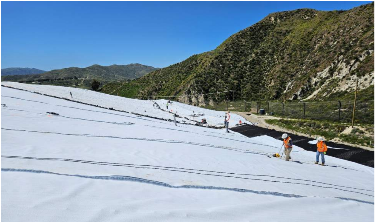
Photo #6 April 10, 2024 Geosynthetic Cover Seaming – North Slope
