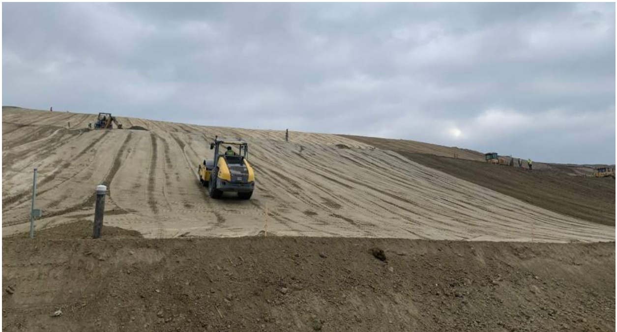
Photo #2 February 29, 2024 Subgrade Preparation – West Slope
