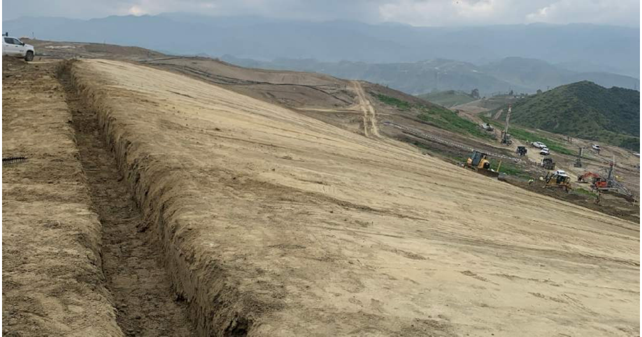
Photo #3 February 29, 2024 Top Deck Anchor Trench – Top of West Slope
