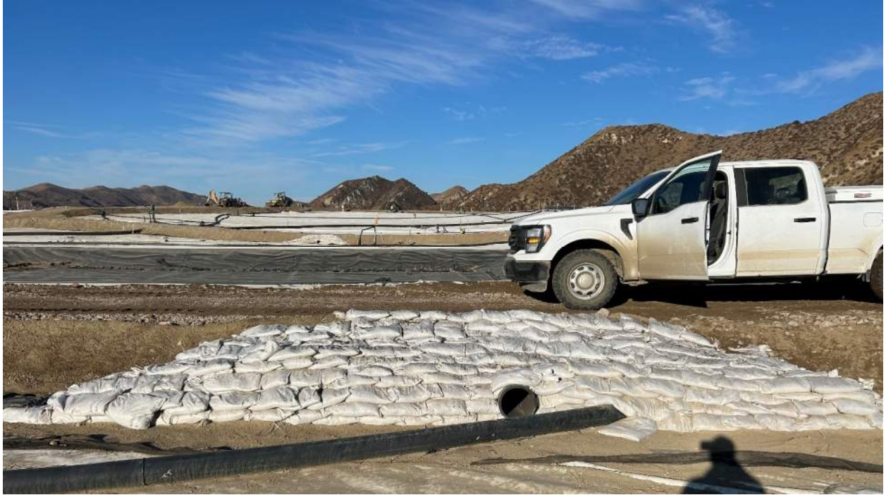
Photo #7 November 1, 2024 Access Road Drainage Crossing – Top Deck
