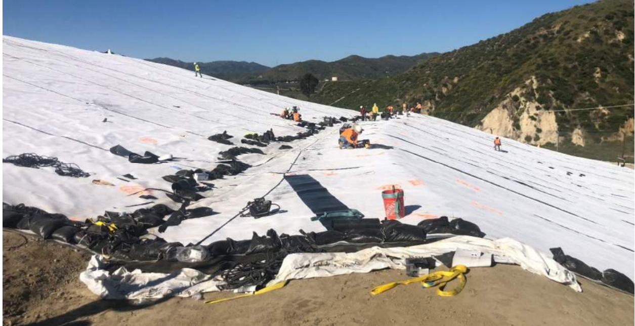
Photo #5 April 10, 2024 Geosynthetic Cover Installation – North Slope
