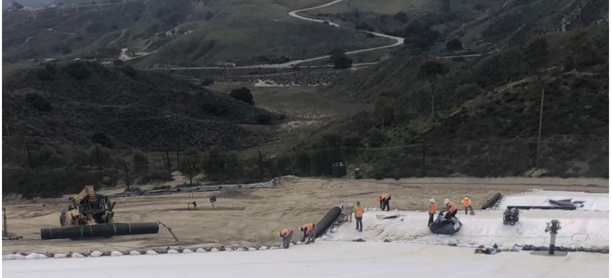
Photo #1 January 31, 2024 Surface Collector Bench Crossing Installation – West Slope
