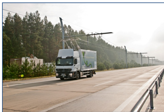
Figure 6 Truck Catenary (Siemens)
