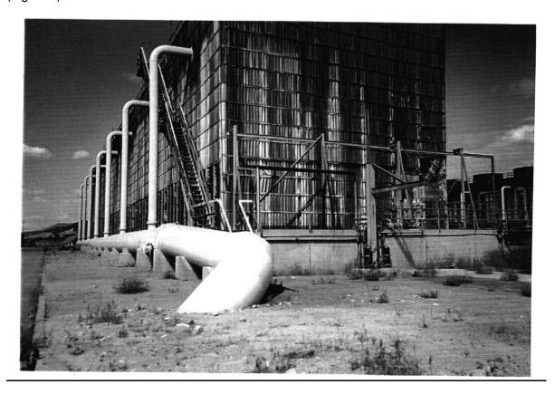
Figure 7. View of Valley Generating Station redwood water cooling tower.
