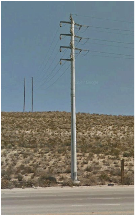
Figure 5: Example TSP Structure
